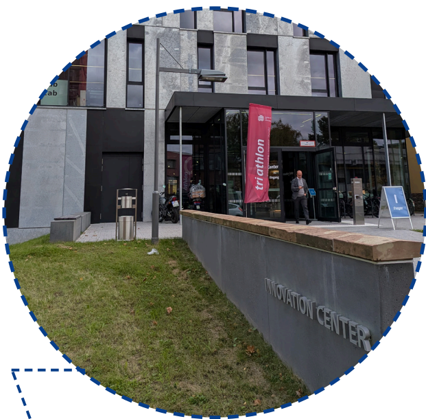
Abb. 47: Innovation Center, Saarbrücken
